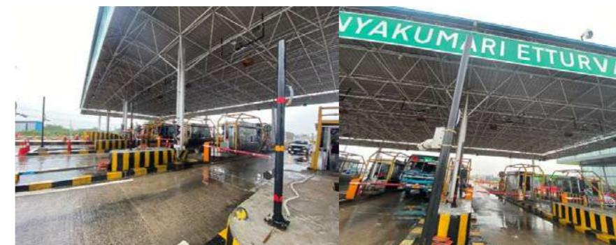
Note: Site visit conducted by EYMSLLP personnel on 18 December 2023
