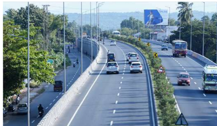
Road furniture provided at curves of the structures
