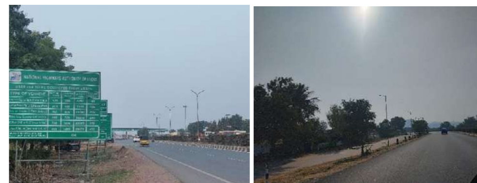
Note: Site visit conducted by EYMSLLP personnel on 20 December 2023
