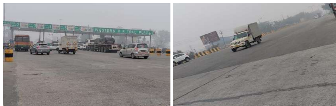
Note: Site visit conducted by EYMSLLP personnel on 22 December 2023
