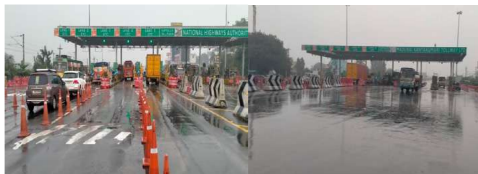
Note: Site visit conducted by EYMSLLP personnel on 18 December 2023
