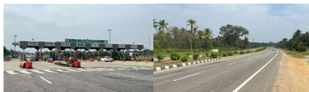
Note: Site visit conducted by EYMBSLLP personnel on 18 December 2023
