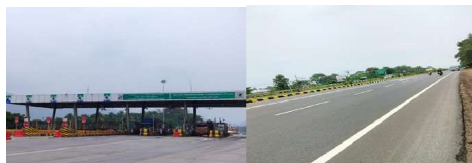
Note: Site visit conducted by EYMBSLLP personnel on 18 December 2023
