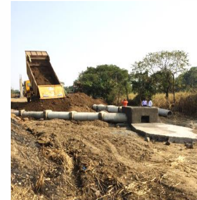
Village infra development
