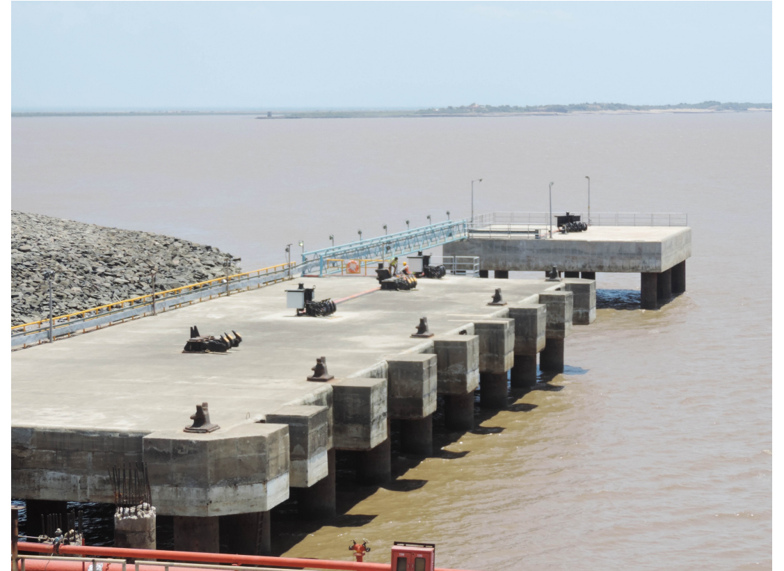
Pipavav Jetty infrastructure upgrade
