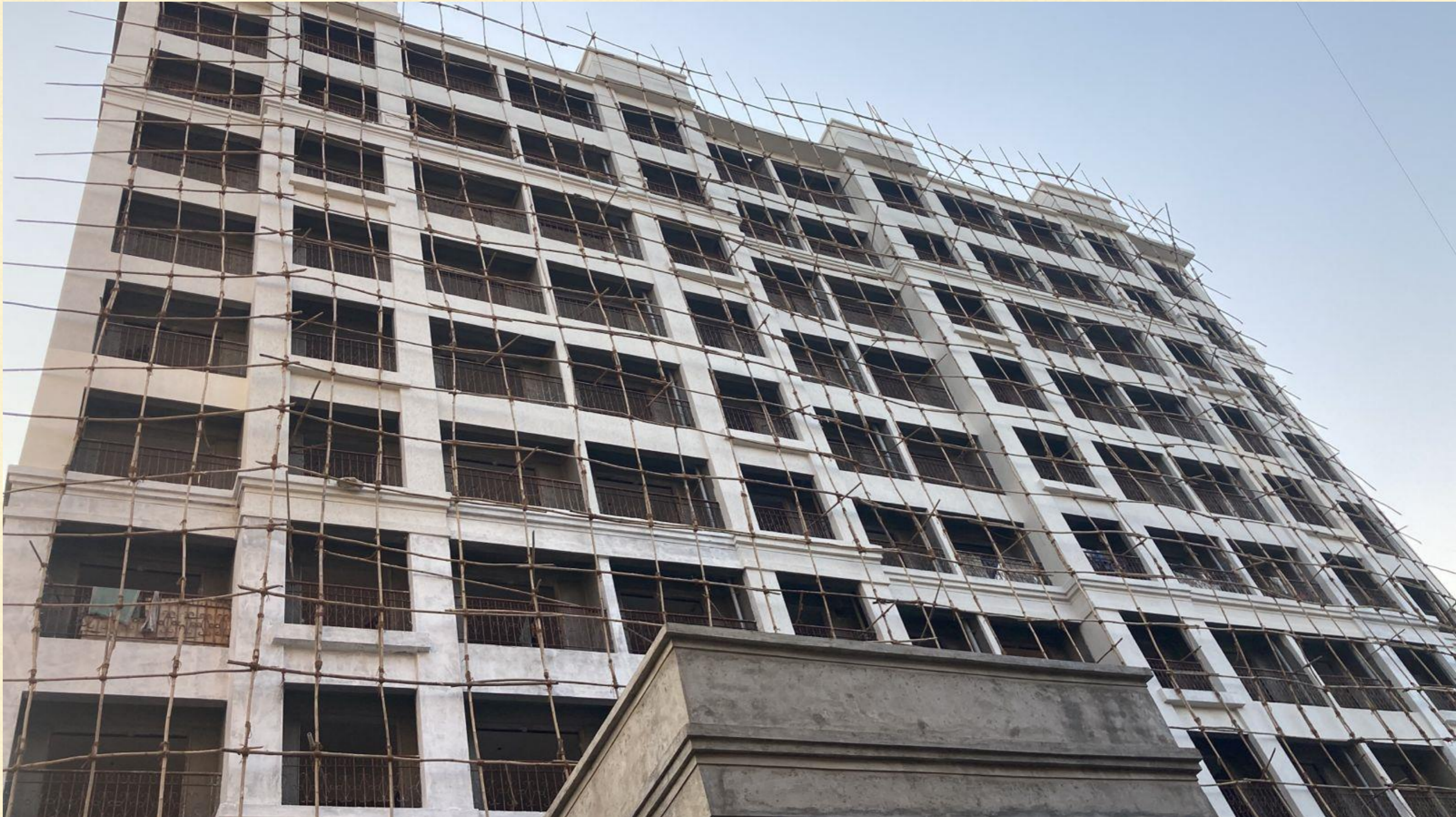
Internal finishing work in progress in Wing-B2
