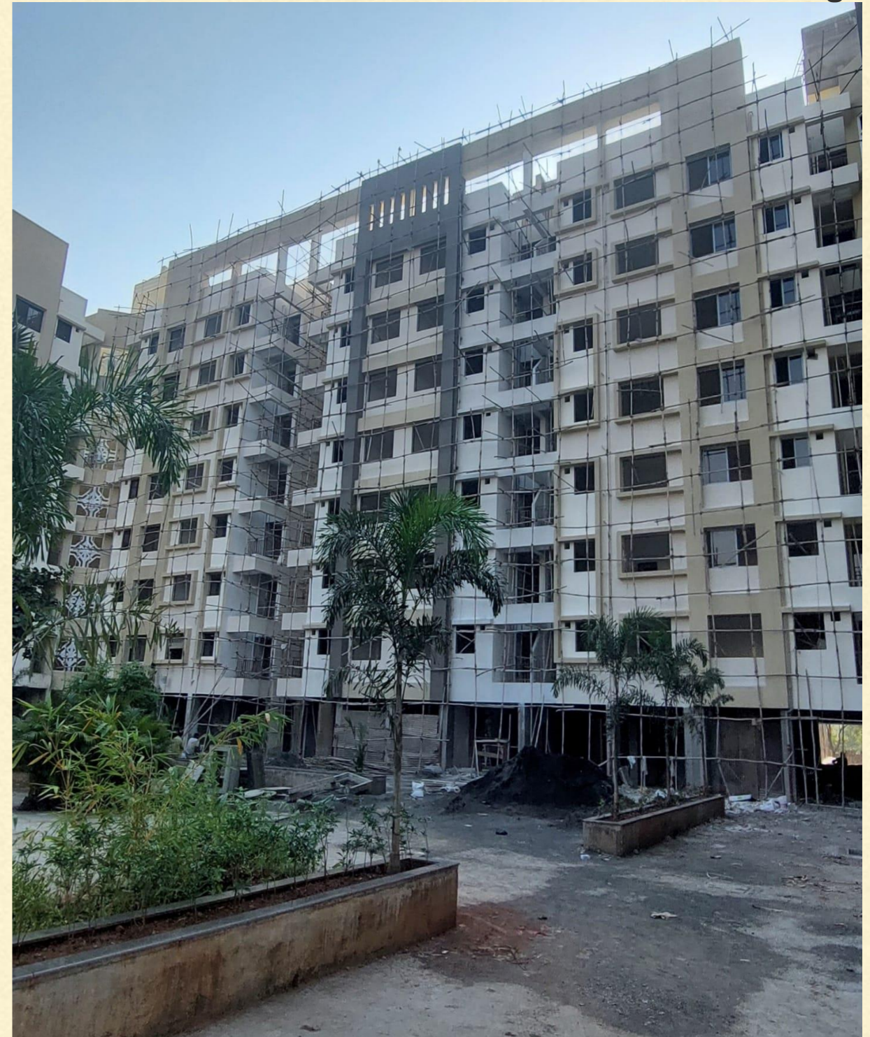
External painting and finishing in progress
