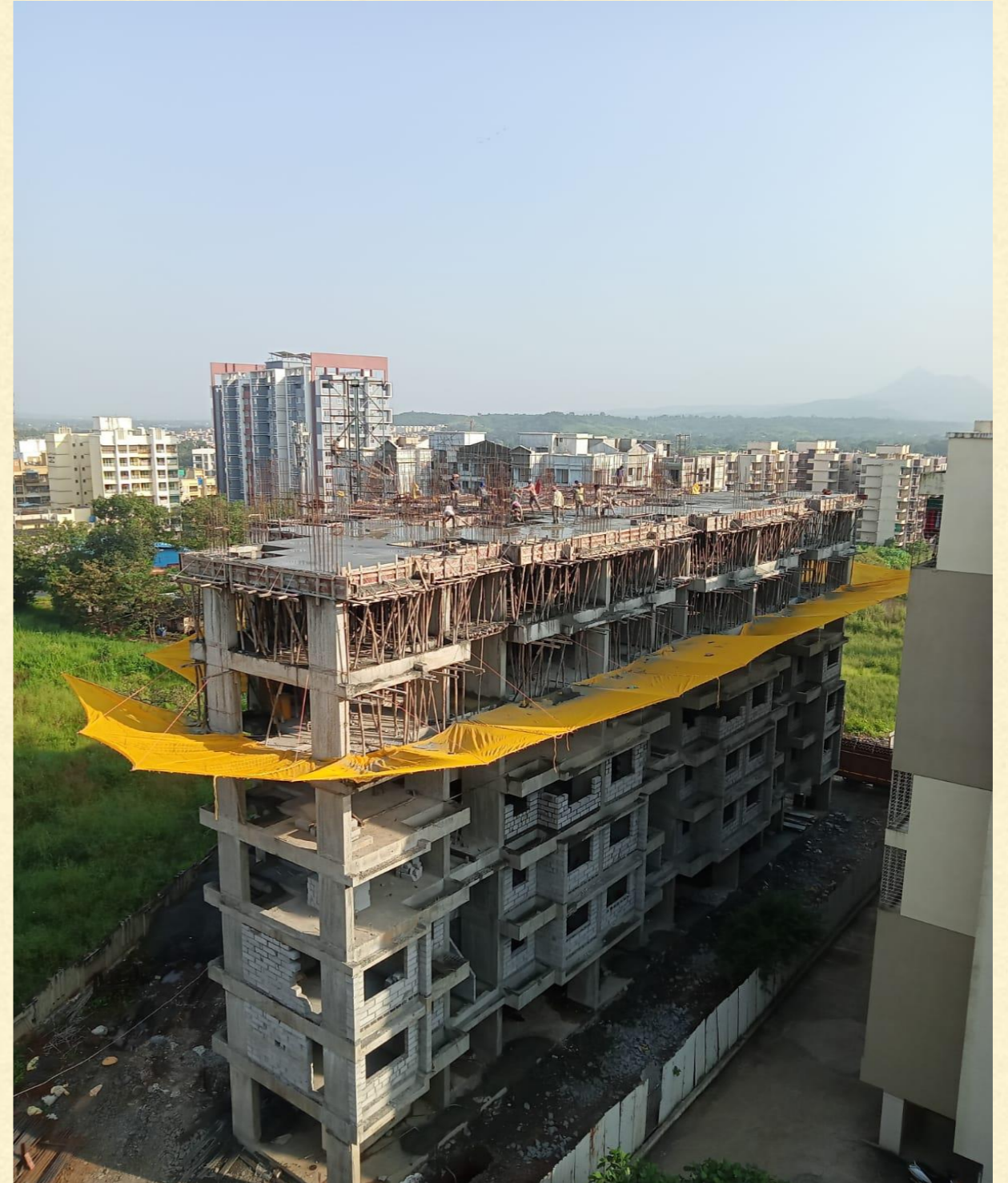
6 th floor completed
