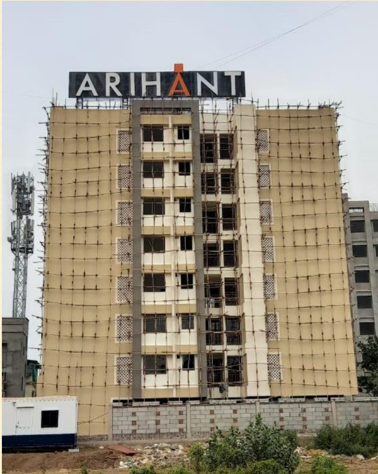
Painting, flooring, firefighting works in progress
