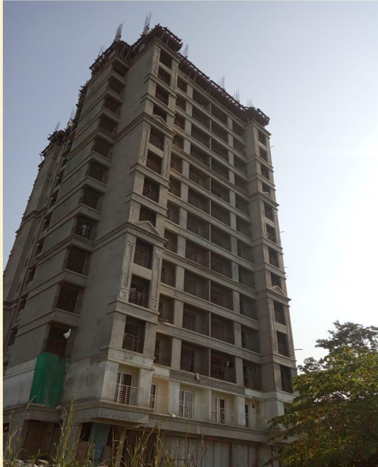
14 th floor completed, internal finishing in progress
