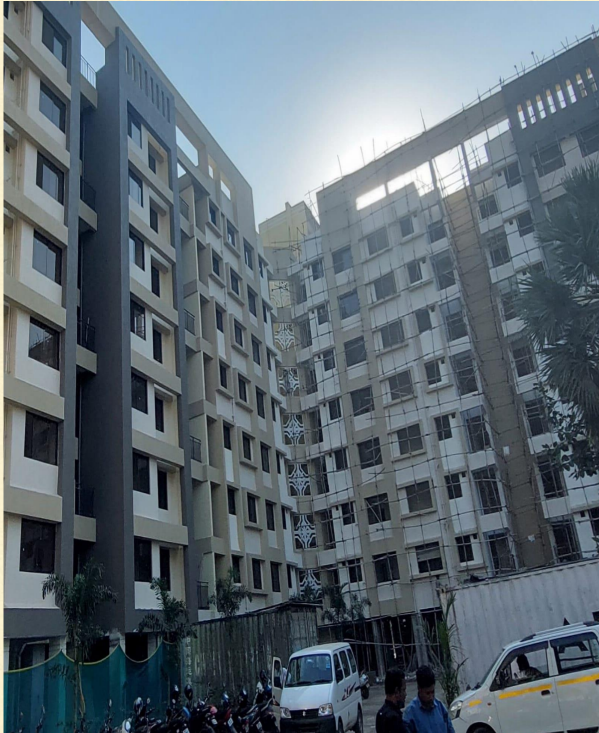
Internal finishing in progress
