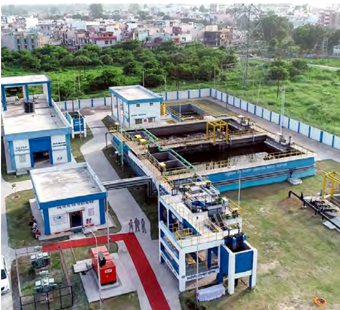
7 MLD Sewage Treatment Plant at BHEL Haridwar
