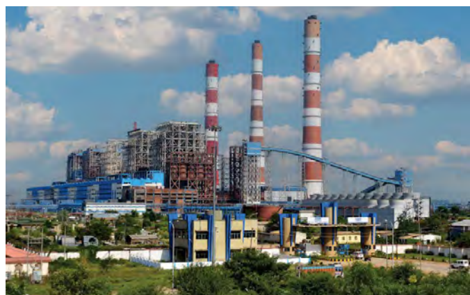
BHEL's first supercritical unit Barh-4 (660 MW) has clocked around 58,009 hours of operation and achieved PLF of 71.2% and OA of 98.5%.
