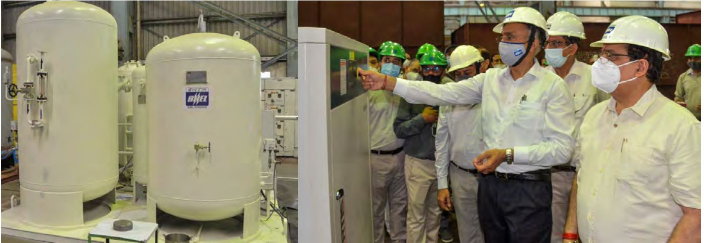
Medical Oxygen Plant at BHEL, Haridwar
