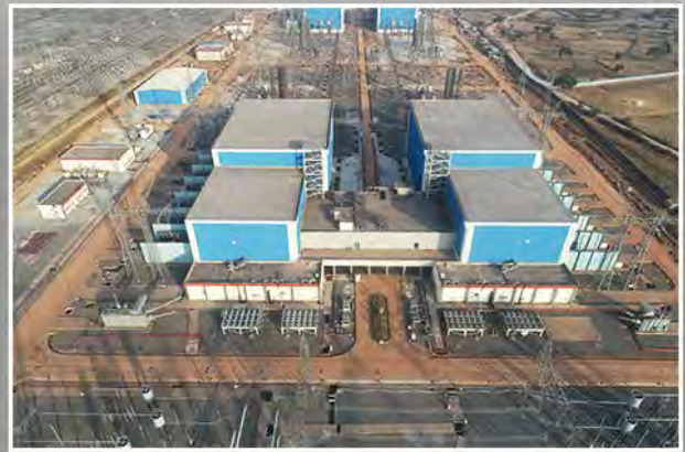
±800 kV, 6,000 MW Ultra High Voltage Direct Current (UHVDC) Link between the Western Region Grid (Raigarh, Chattisgarh) and the Southern Region Grid (Pugalur, Tamil Nadu) successfully implemented by BHEL.
