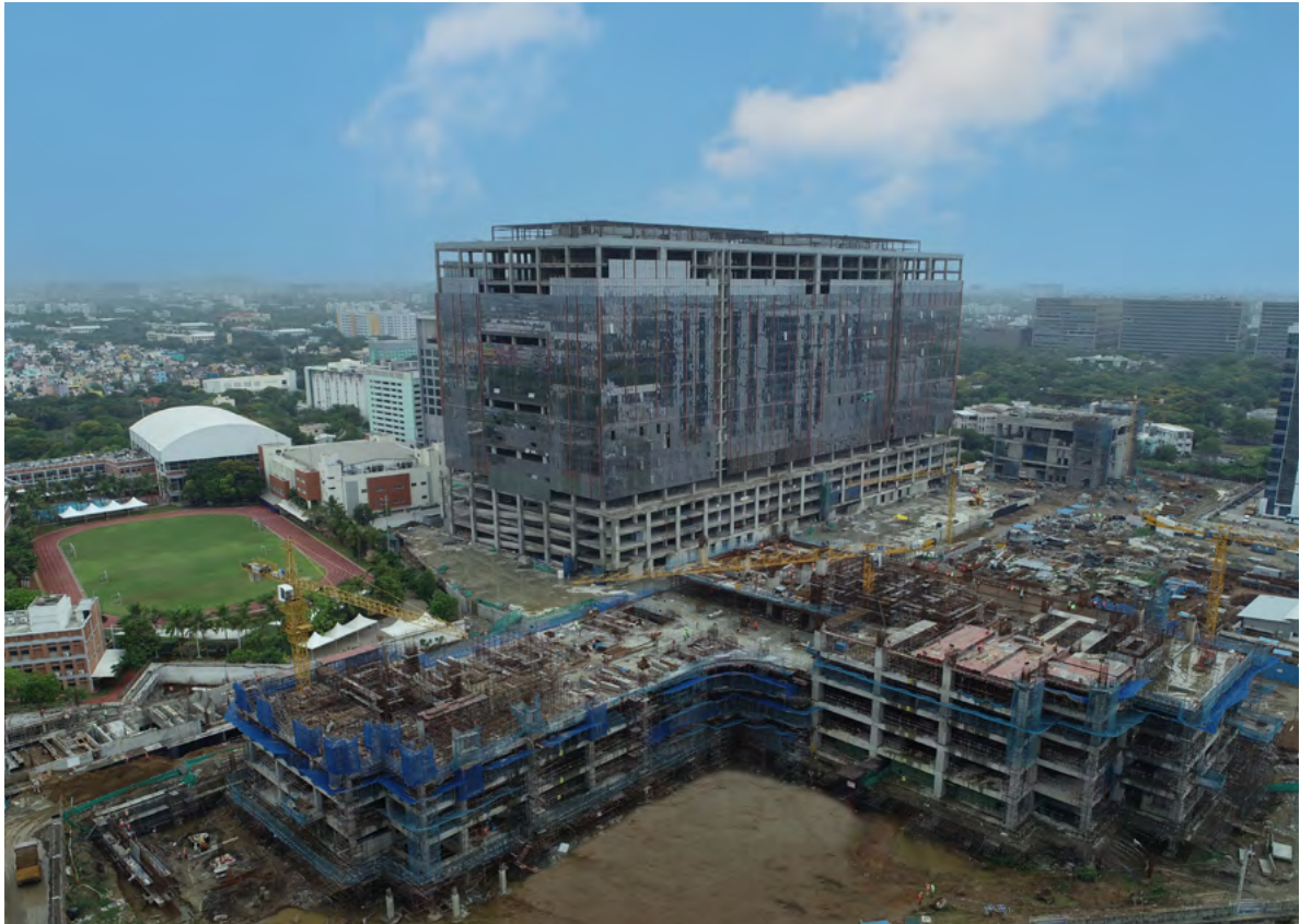
DLF Downtown under development in Chennai
