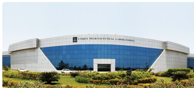
State-of-the-art Formulations manufacturing facility at Panoli, Gujarat
