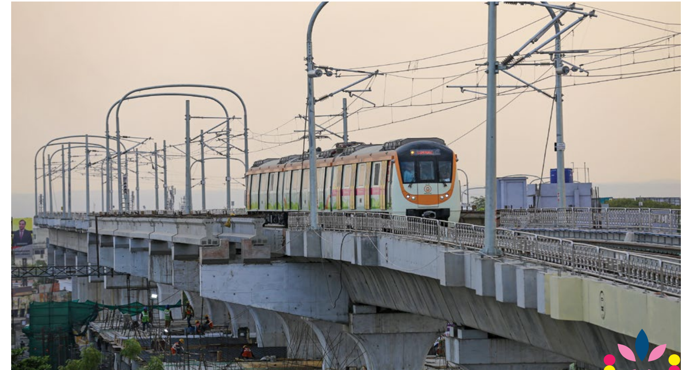
Elevated Stations for Nagpur Metro, painted by AP-PPG coatings (EPC - ITD Cementation)
