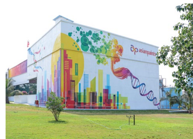
Research & Technology Centre at Turbhe, Navi Mumbai
