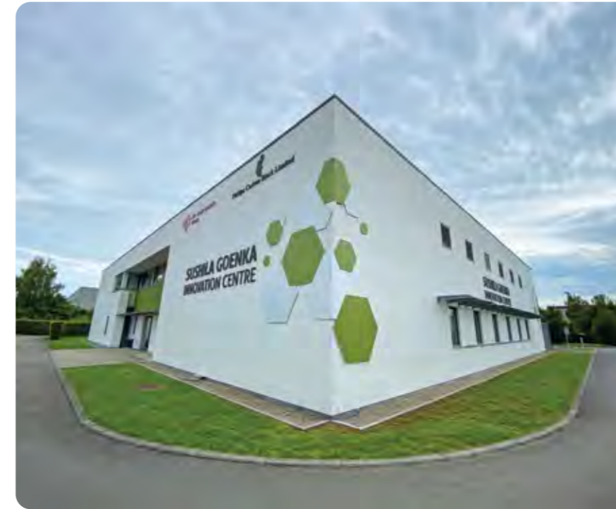
Outer view of Sushila Goenka Innovation Centre, Ghislenghien, Belgium
