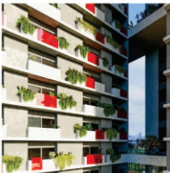
Green Building Façade up-close
