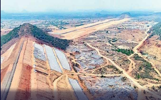
400/11kV AIS substation for powering lift irrigation
