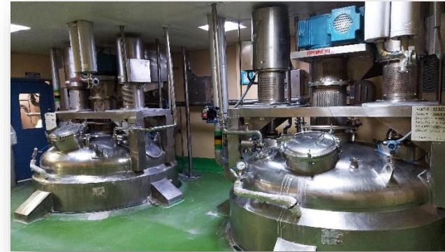
Main Mixing Tank
