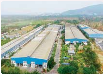
VIZIENAGARAM Near Visakhapatnam, Andhra Pradesh Product line: 2V/12V-AGM VRLA & Tubular Gel
