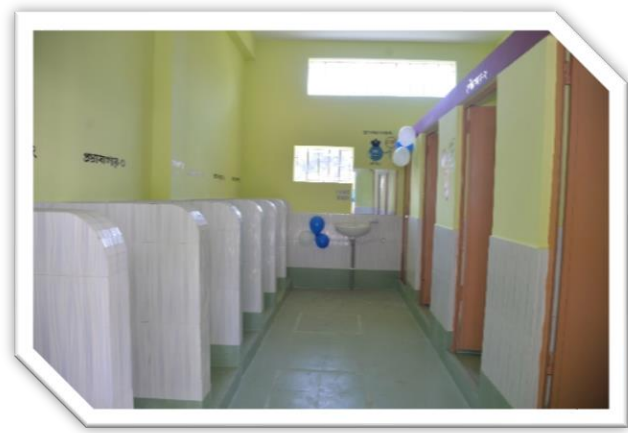
Toilets Constructed in Schools- West Bengal & Haryana
