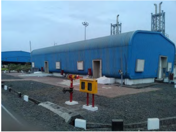
CS - 8 Electric Sub Station
