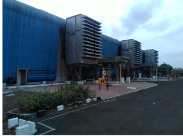
CS - 8 Compressor House
