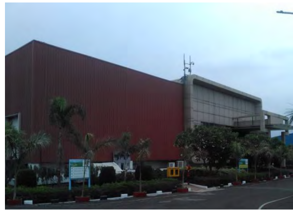
CS - 8 Local Control Room Building
