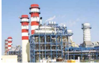
2X157 MW GT POWER PLANT, LIBYA (COMPLETED)
