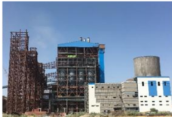
2X660 MW STPP, BOILER , ESP, STRUCTURE & STG U#7&8, SURATGARH, BHEL
