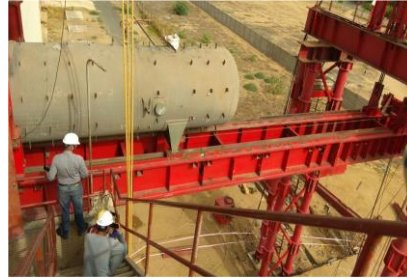
HP HEATER REPLACEMENT 800MW ,CGPL MUNDRA2
