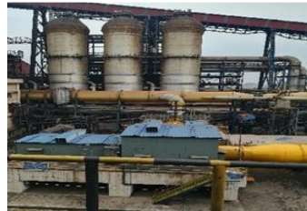
BLAST FURNACE, STEEL PLANT WORK, JSPL, ANGUL
