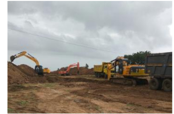
KALWESHWARAM CANAL PROJECT, 54 KM RAMAYAMPET
