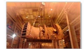
3X 126 MW, KHOMS, GECOL, LIBYA TOP CASING LIFTING
