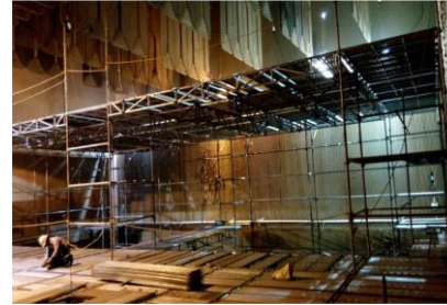
CUPLOCK SCAFFOLDING ERECTION 800MW,MUNDRA
