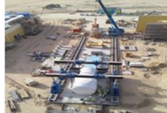
1519 MW FADHILI CCPP, SAUDI ARABIA GTG,STG & BOP INSTALLATION
