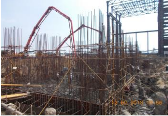
1X800 MW TPSS , CIVIL, STRUCTURAL WORKS, NORTH CHENNAI, BHEL
