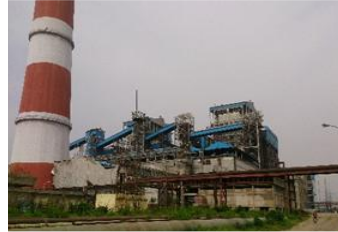
2X500 MW STPP,BOILER, ESP STG, VINDHYACHAL, BHEL (COMPLETED)
