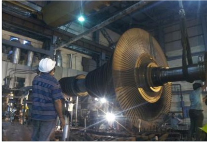
CAPITAL OVERHAULING OF TURBINE 63MW, SV POWER , KORBA - ROTOR LIFTING-3
