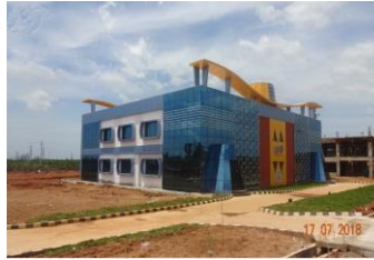
INFRASTRUCTURE DEVELOPMENT WORK, AP MEDI TECH ZONE, VIZAG
