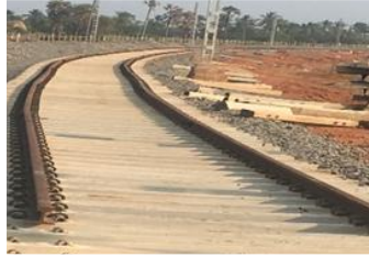
GDV-MTM 37 ,DOUBLING & ELECTRIFICATION WORKS , RVNL
