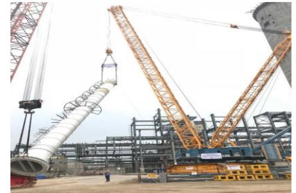
UREA REACTOR TANK INSTALLATION AT RAMAGAUNDAM, TELANGANA
