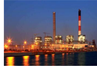
BOILER, ESP, TG AUXILIARIES, UMPP 800 MW, GUJARAT, TATA POWER (COMPLETED)
