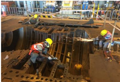
MAIN TURBINE OVERHAULING ,660 MW KAWAI
