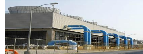
Infrastructure Construction (Civil)
