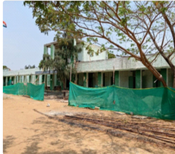
Govt. School - Renovation
