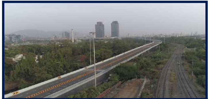
Thane Belapur Flyover
