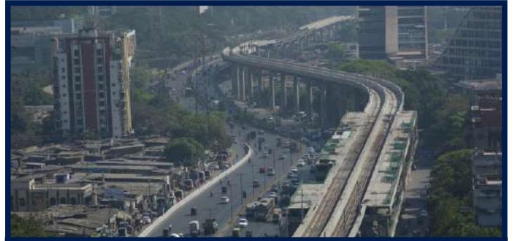
Mumbai Metro - Line 7
