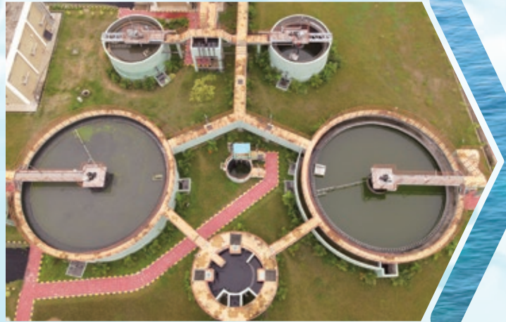
Cuttack 2 WTP, Odisha
