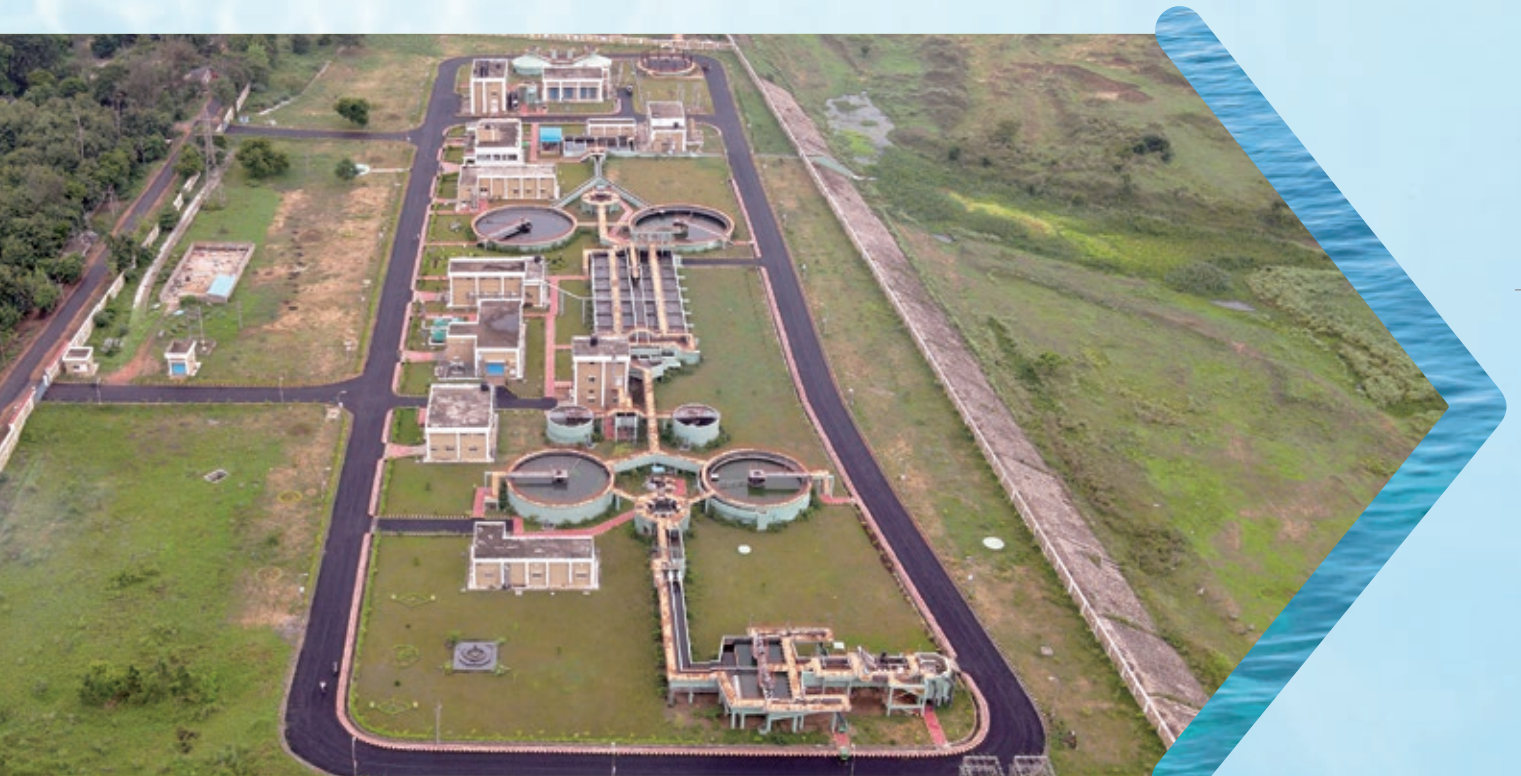
Cuttack 02 WWTP, India
