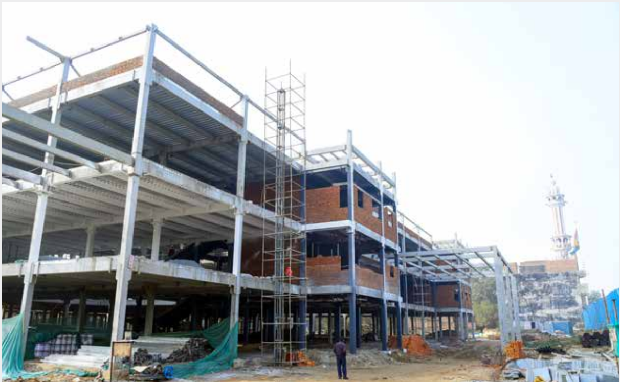
Area of 1.5mn square feet being built using 100% Apollo Column Tubes
