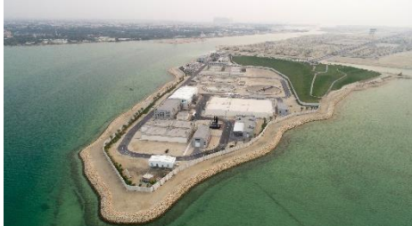
Al Madina Al Shamaliya 40 MLD Sewage Treatment Plant, Bahrain Awarded Wastewater Project of the Year at Global Water Awards, 2019
