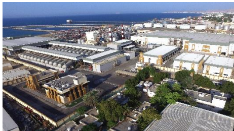
191 MLD SWRO (Desalination) Plant, Al Gubrah, Oman Largest desalination plant in the country of Oman
