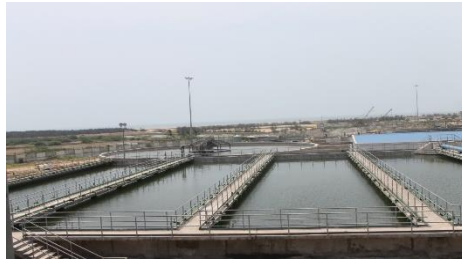
54 MLD Effluent Treatment and recycling plant, for Indian Oil Corporation Limited, Paradip, Odisha, India India's largest industrial water recycling plant
