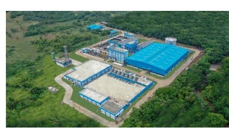
45 MLD Koyambedu TTRO Recycle Reuse Plant, Chennai, India One of the largest and technologically most advanced water reuse plants in India ensuring Chennai's Water security
