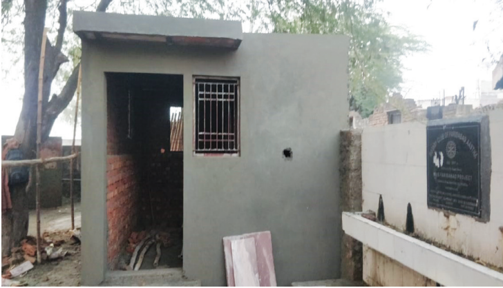
Toilet Construction at Govt. School, Faridabad
