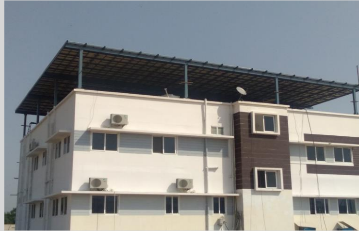
ROOFING WITH THE ATUM PANELS
