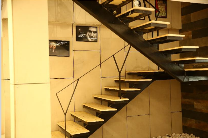
Mezzanine Flooring with V-Boards
