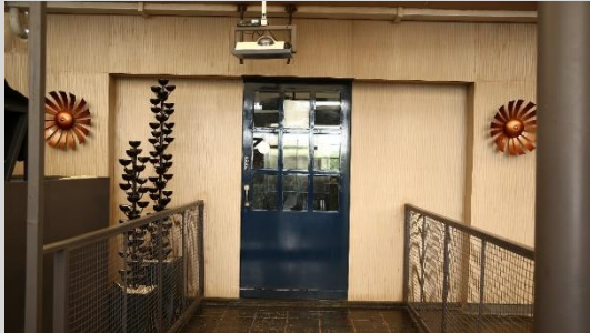
Wall Paneling with V-Boards
