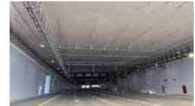
Mina Zayed Tunnel - Abu Dhabi
