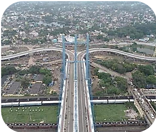
Road Over Bridge at Burdwan - Plasticated LRPC
