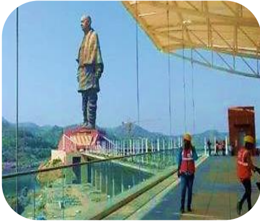
Sardar Vallabhbhai Patel Statue, Gujarat - Pavilion roof structure supporting cables
