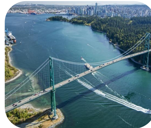
Lions Gate Vancouver, Canada - Supporting locked coil
