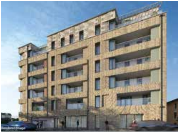
Southhall Men's Working Club, Southhall
