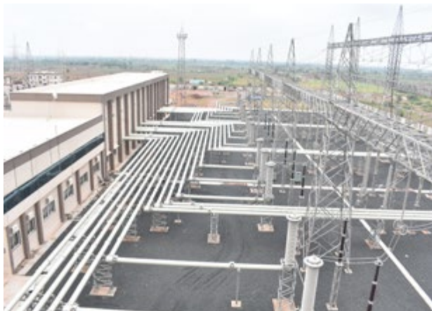
400/220kV GIS for GETCO at Shapar
