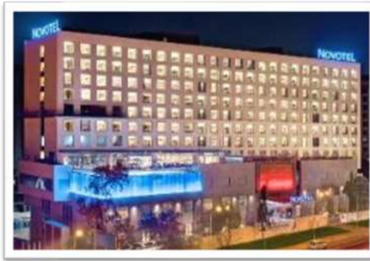
Addition of 88 rooms at Novotel Pune
