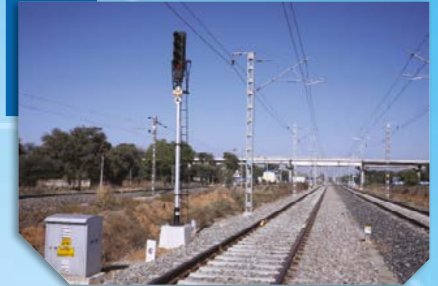
Main Signal, Apparatus Case & TLJB of MSDAC
