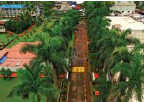
Sudarshan Chemical Industries, Plant View
