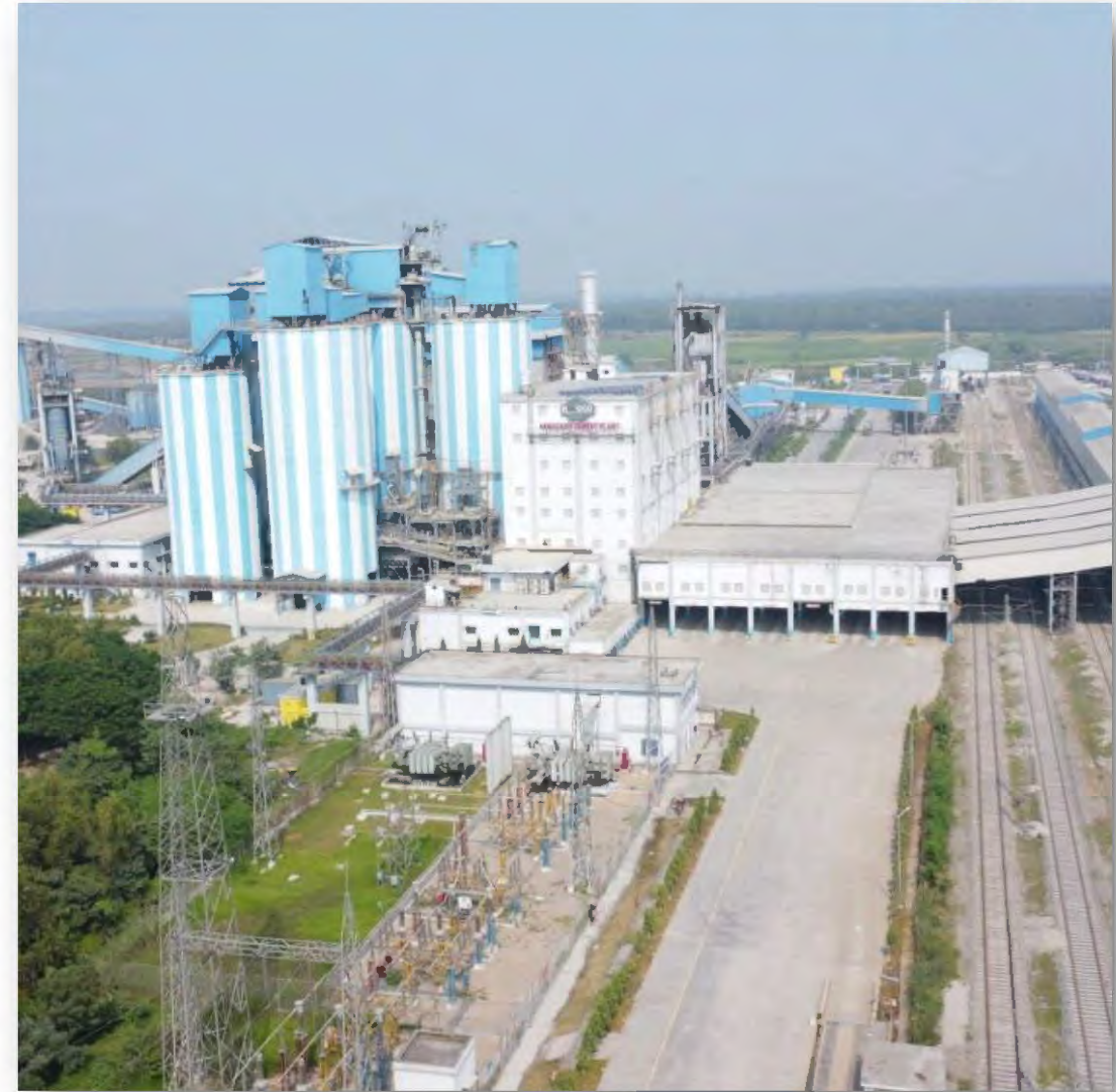
Panagarh Cement Plant
