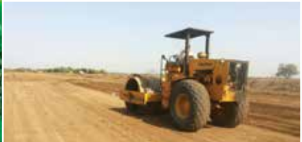
Work in progress at embankment top layer
