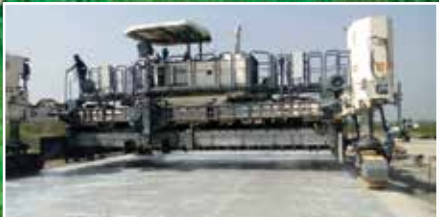
Pavement Quality Concrete (PQC)
