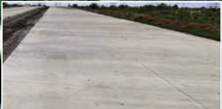
Finish layer of Highway
