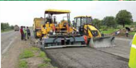
Dry Lean Concrete (DLC)
