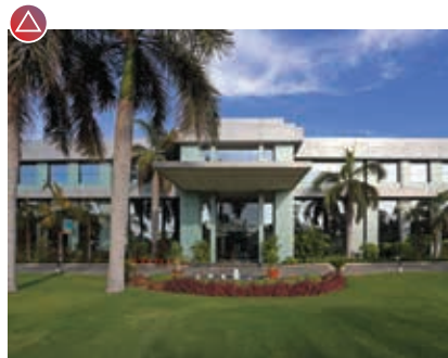
HEIL Changodar Plant
