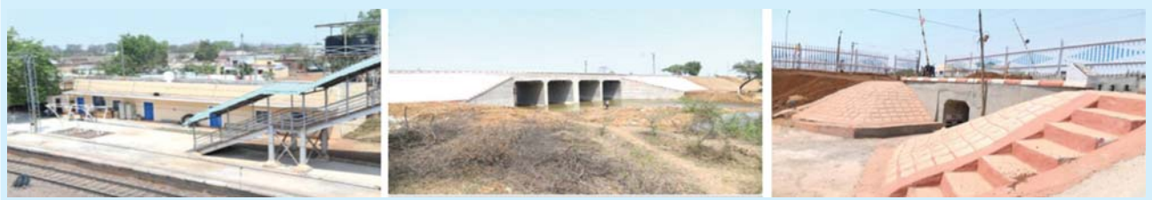
Commissioning of Doubling with Electrification of Arangmahandi-Lakholi Section on 5th Aug, 2021.
