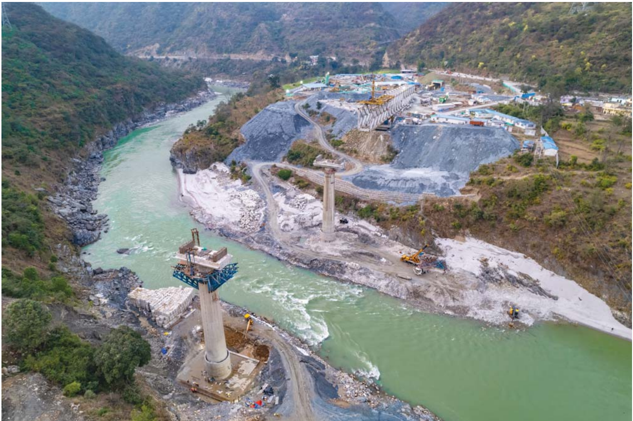
Successful completion of substructure works of Rail Bridge no 8 in connection with ongoing new BG Rail Line Rishikesh- Karnaprayag Project https://youtube/AwXC04aL89s
