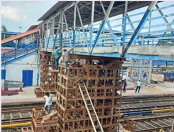
Raising of FOB Over 3 Tracks And 2 Platforms at New Bongaigaon
