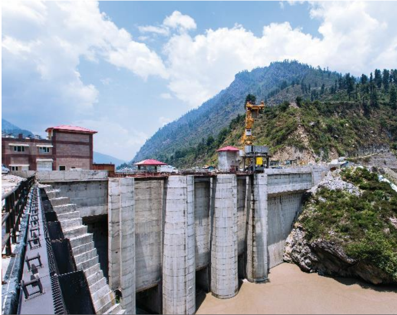
Parbati Hydro Electro Project (800 MW)
