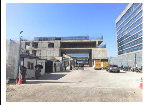
External view of the subject property (SP)
