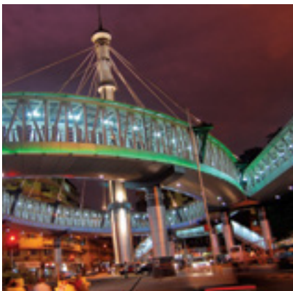
Grant road Skywalk
