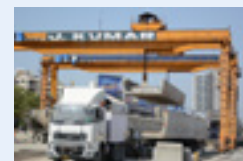
Casting yard (Elevated metro)
