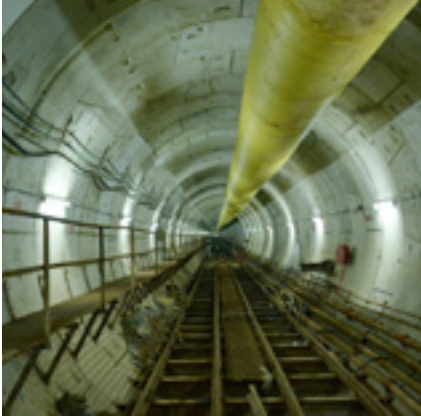
Mumbai Metro Line 3
