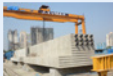
Casting yard (Underground metro)
