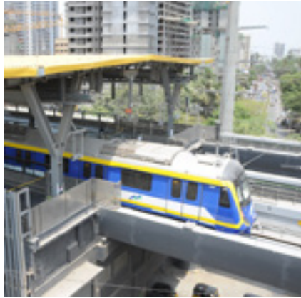
Mumbai Metro Line 2A
