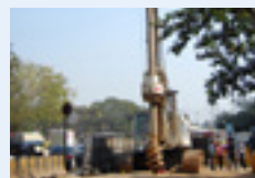
Hydraulic piling rig
