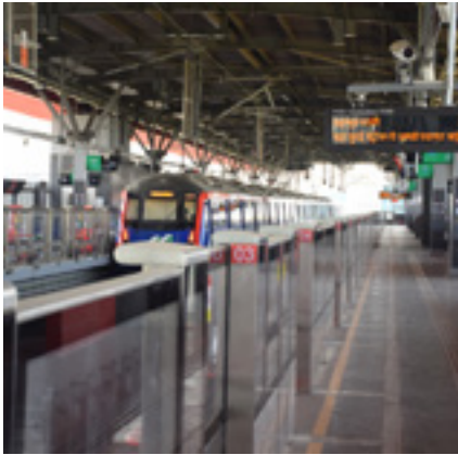
Mumbai Metro Line 7
