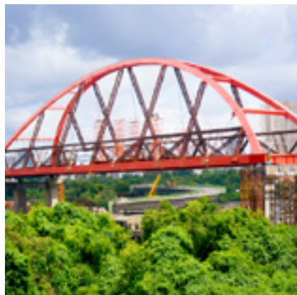
Kalwa Bridge Thane
