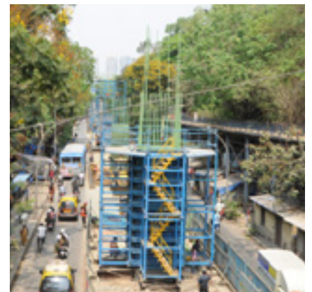
Sewri Worli Elevated
