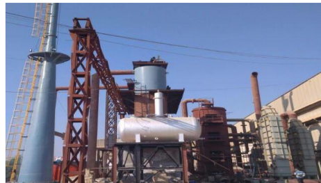
Kisan Phosphates, Haryana: Fertilisers Plant
