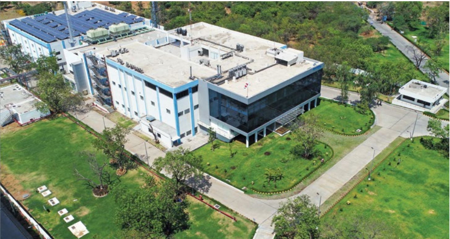
Oncology Injectable and OSD plant
