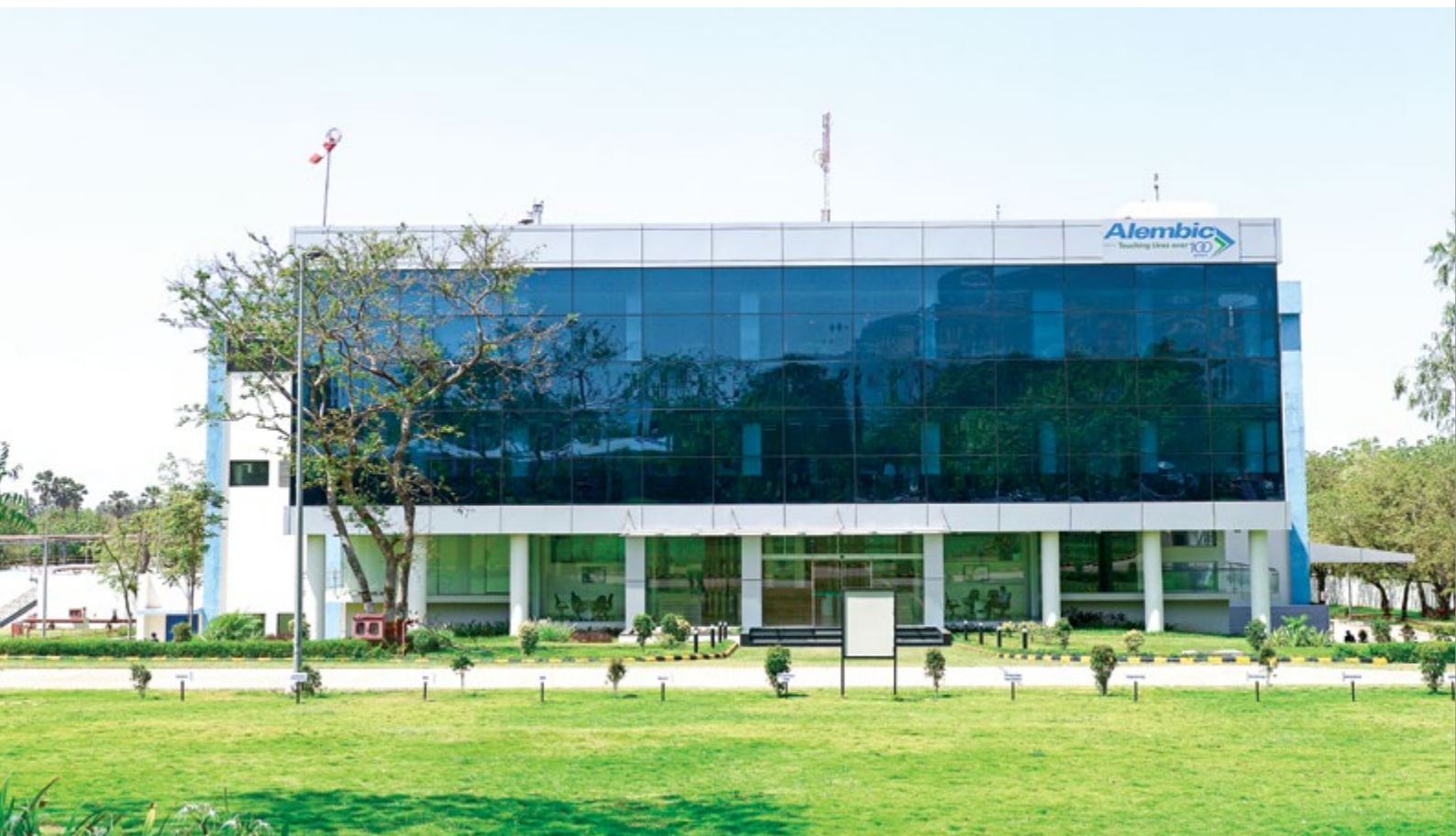
Oncology injectable and OSD plant (F2), Panelav
