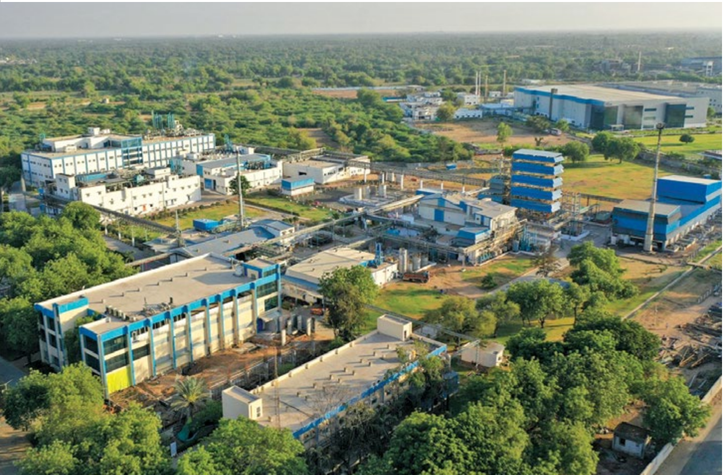
API plant, Karkhadi
