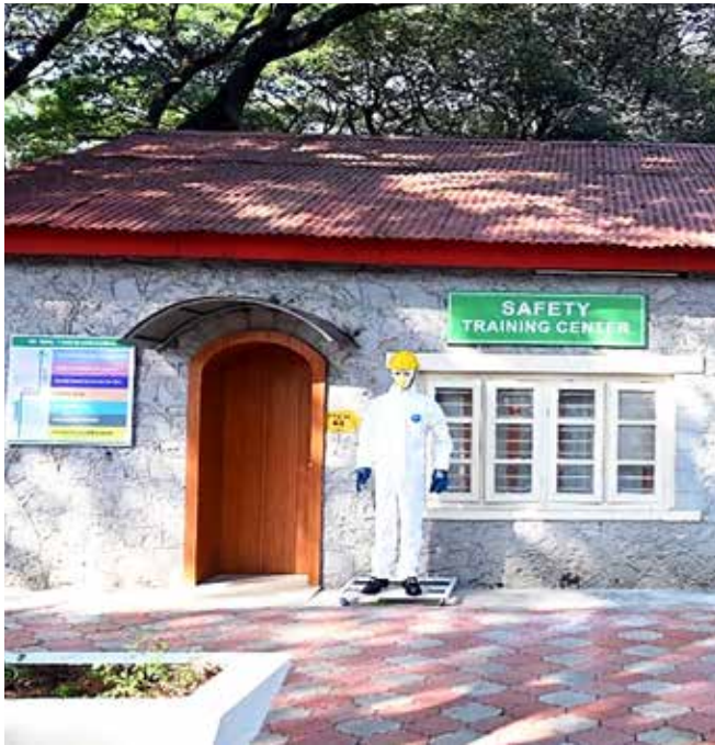
Safety Training Center at Kirloskarvadi Plant
