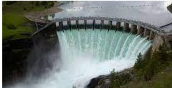
Kopili Hydro Electric Project, Assam
