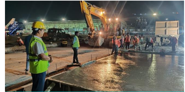
International Airport Taxiway Project, Chennai
