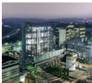
Our ATBS plant at Lote, Maharashtra
