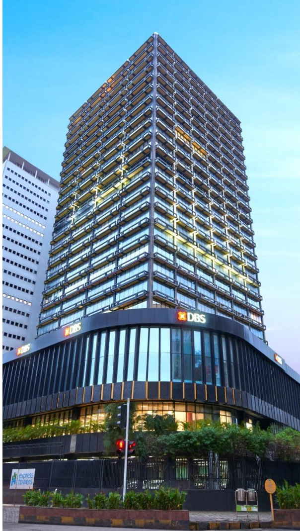
Express Towers Mumbai (0.5 msf)
