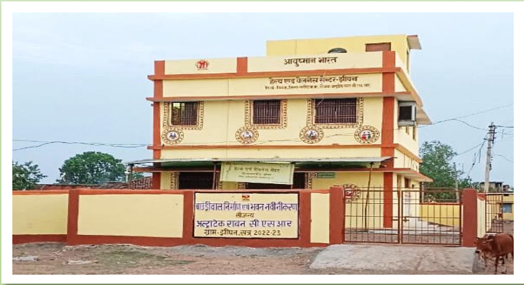
Village infrastructures were strengthened in nearby villages at various unit locations
