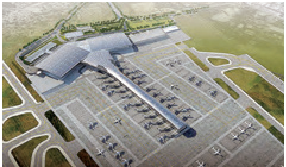
| HVAC services for Delhi International Airport
