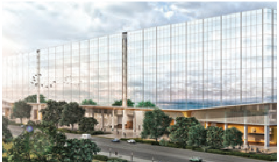
| MEP services including GIS substation at DLF Cyber Park, Gurugram
