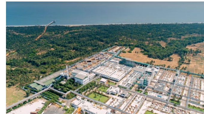
Off-the-ground effluent treatment plant
