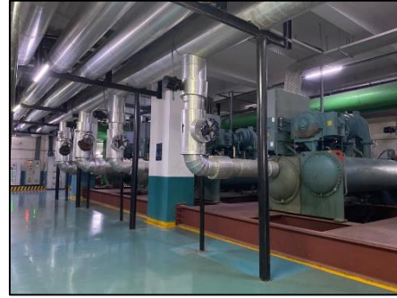
Internal View of Plant Room Tower 4,5,6
