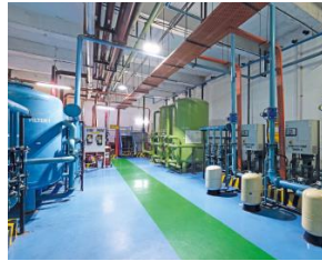
100% of the wastewater treated and reused onsite
