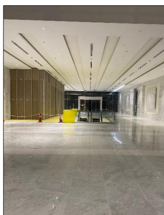
Internal View of Tower 11
