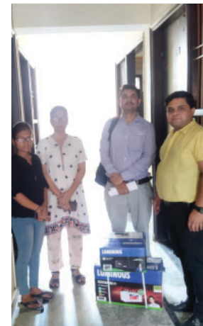
Donated Inverter system for power backup
