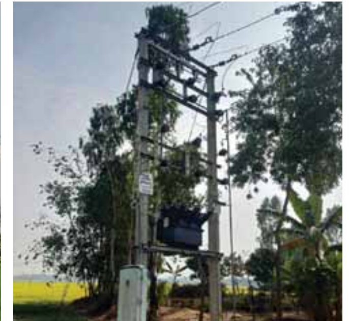
Feeder Separation Projects
