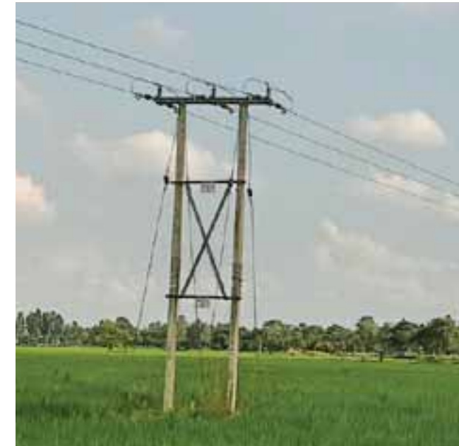
Rural Electrification Works
