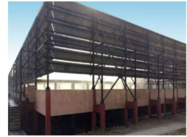
Mist Cooling System
